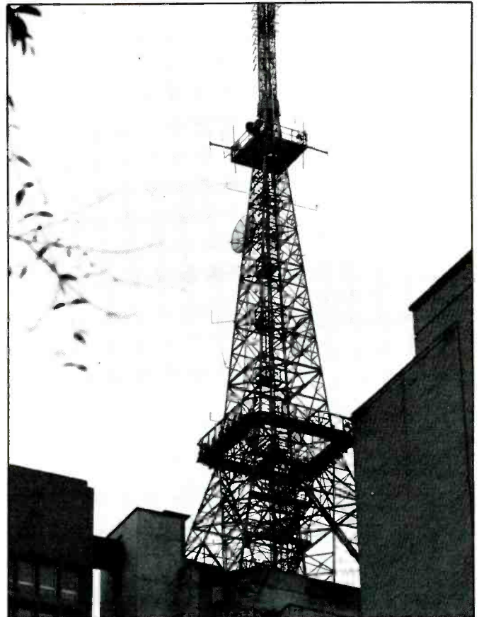
This is the Sao Paulo TV Channel 7 tower, which piggybacks many other antennas, including one for ham TV. (Courtesy Helio Soares, Brazil.)
