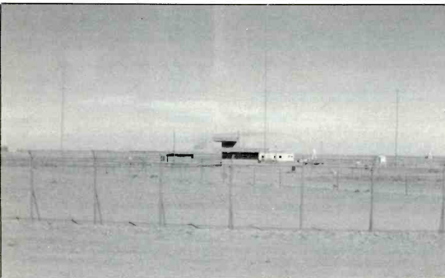
One of the microwave towers in Al-Qaisumah. Thanks for photo go to Kevin Tubbs, Saudi Arabia.
